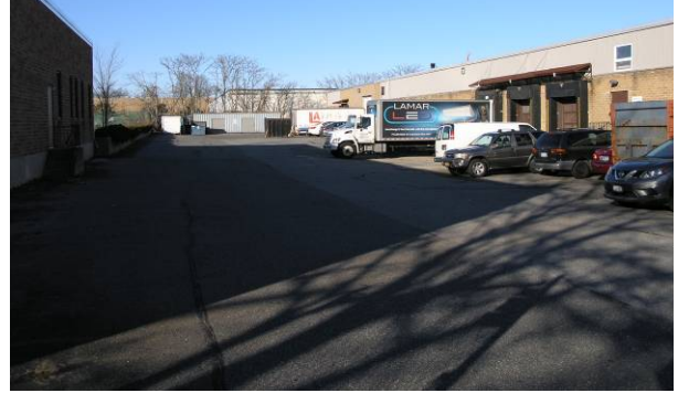
West Side of Building
