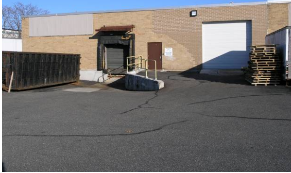
West Side of Building
