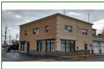
271 Central Ave Bethpage, NY 11714
