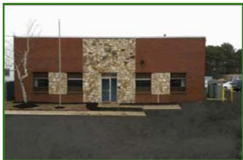
1605 Sycamore Ave (Yard) Bohemia, NY 11716
