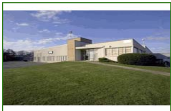
92 Central Ave Rear Sec Unit B Farmingdale, NY 11735
