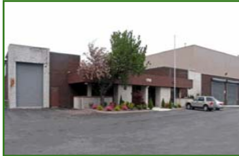
1765 Expressway Dr N Hauppauge, NY 11788
