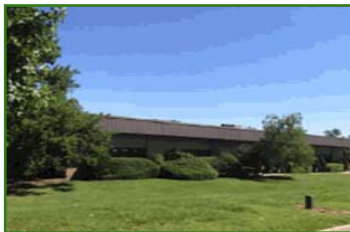
175 Engineers Rd Hauppauge, NY 11788
