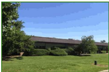
175 Engineers Rd Hauppauge, NY 11788
