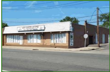
920 Wellwood Ave Lindenhurst, NY 11757
