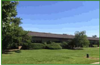
175 Engineers Rd Hauppauge, NY 11788
