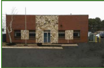
1605 Sycamore Ave Bohemia, NY 11716
