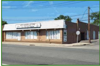
920 Wellwood Ave Lindenhurst, NY 11757
