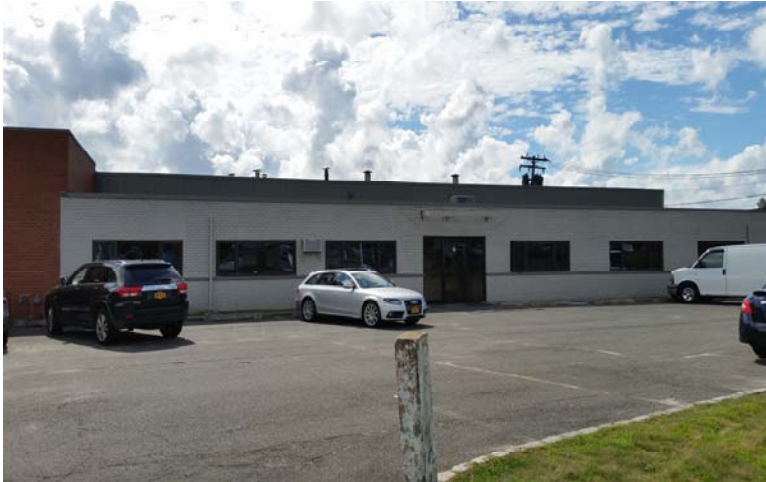
FRONT OF BUILDING
